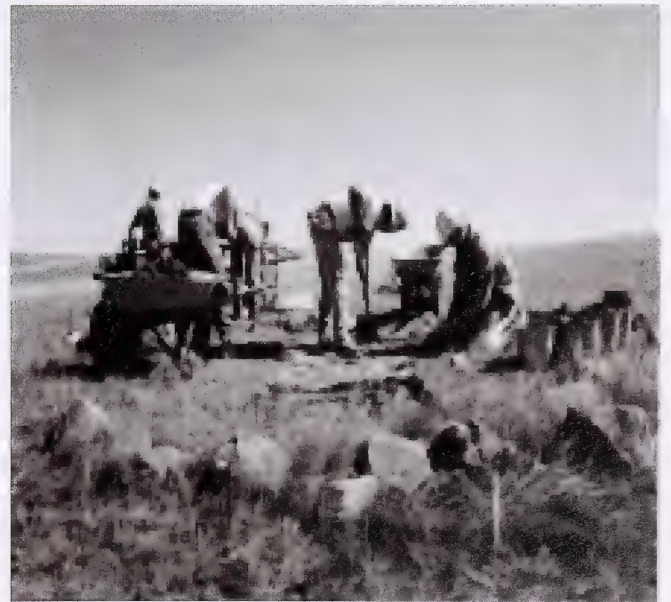
Photo 21 Historic resource impact mitigation
